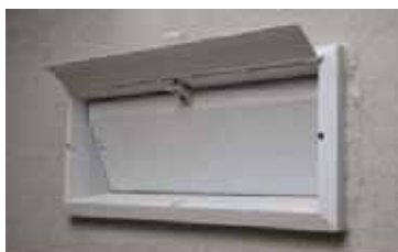
Reduce/close the air inlet when vaccinating
